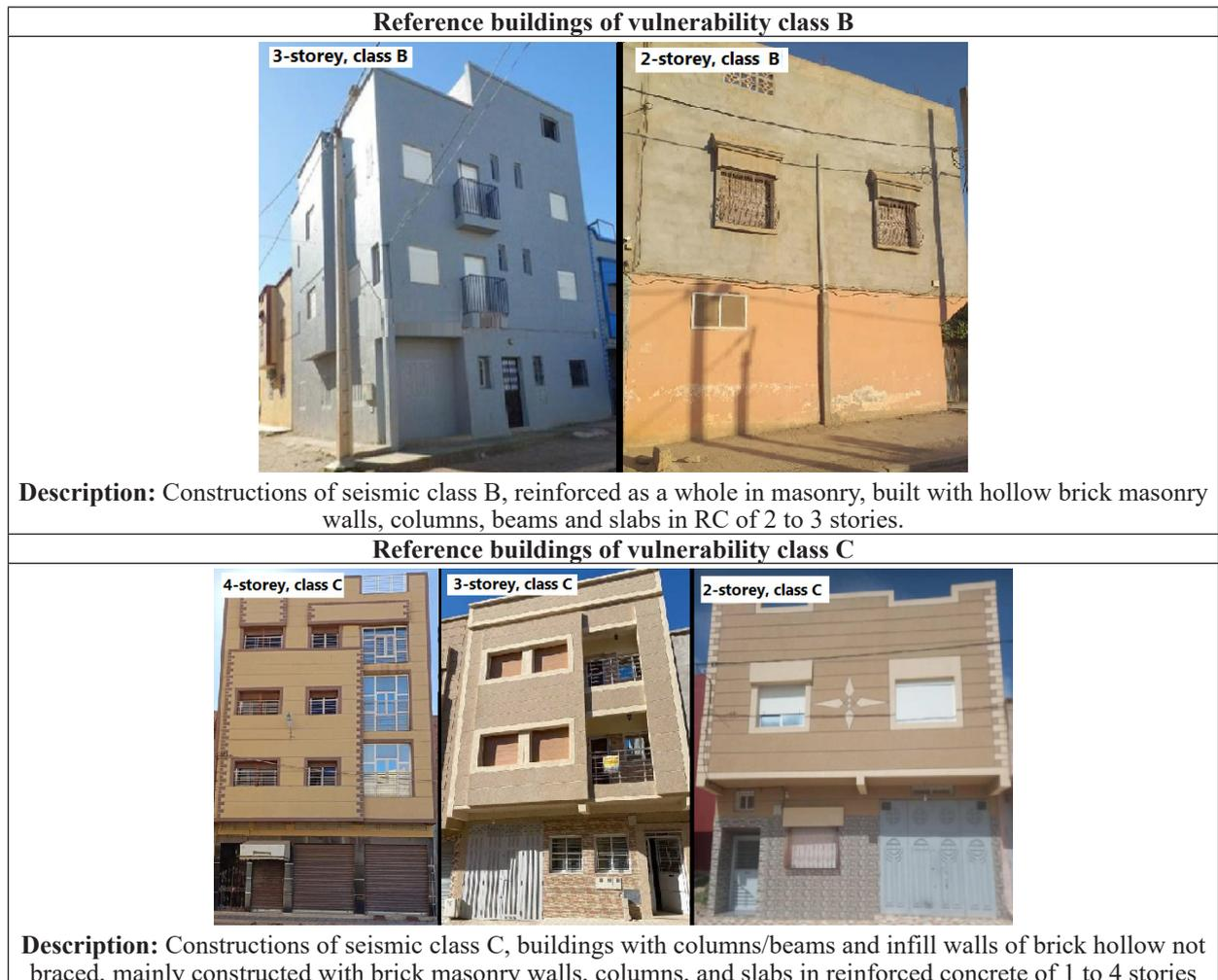
Figure 7. Illustration of the classification of buildings selected for the analysis by the deterministic method.
